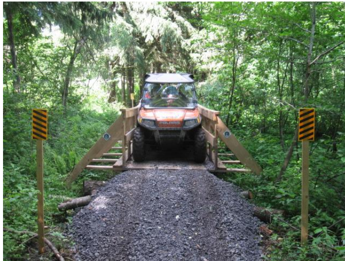
BRIDGE PLACEMENT WITH RAILS
